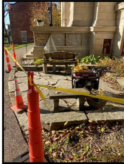
Entry Staircase – North Wall – Stone Replacement
