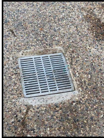
North Side (north) – Repaired Sidewalk Drain
