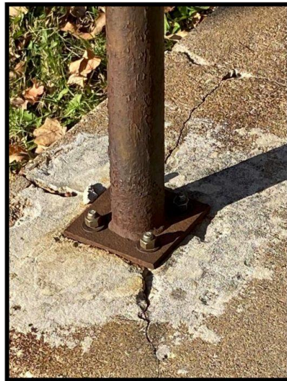
Example of New Base Plate and Expansion Anchors
