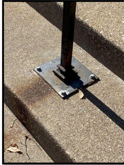
Entry Staircase – New Base Connection
