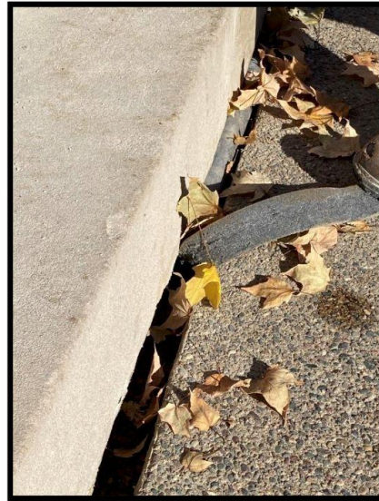
Entry Staircase with Pea Gravel at Base of Joint
