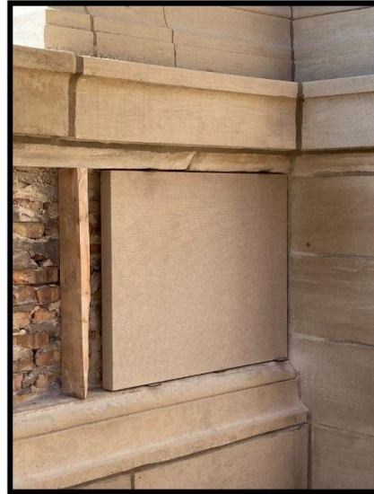
Entry Staircase – North Wall - New Stone Piece
