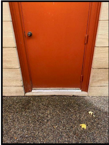
North Side – Exterior Closet – New Threshold
