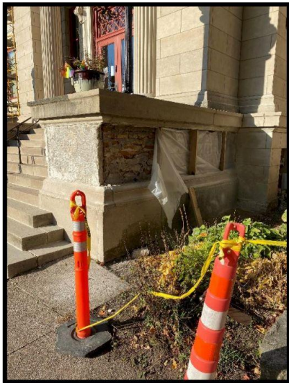
Entry Staircase – North Wall – Stone Replacement
