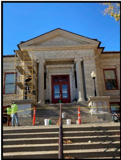
Front Façade (east side) – Joints Repaired
