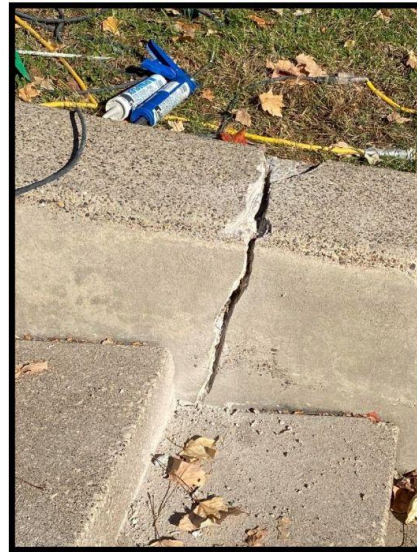
Entry Staircase – Routing Out Crack for Sealant/Caulk
