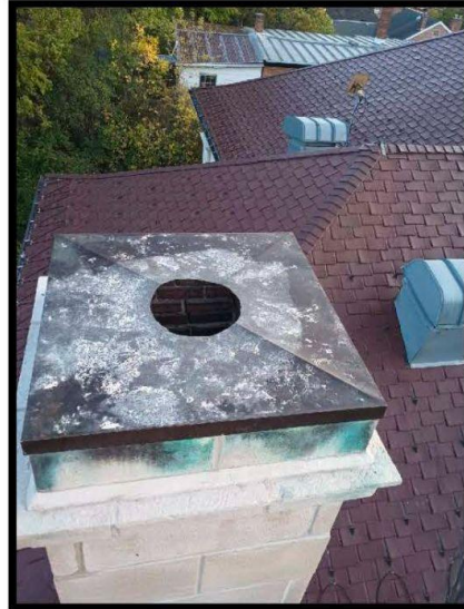
Chimney – Copper Cap with Hole
