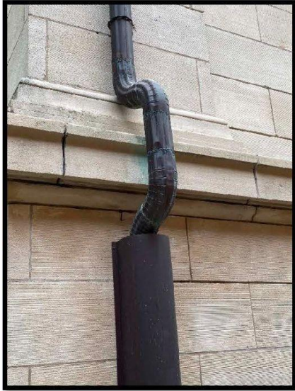
Stonework with Ground Out Joints and Power Washed
