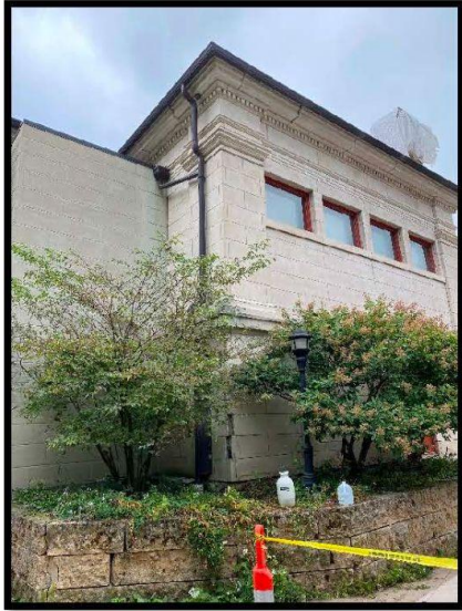
Corner Stonework Deterioration
