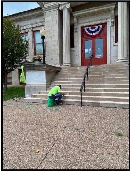
Entry Steps – Sealant/Caulk Removal
