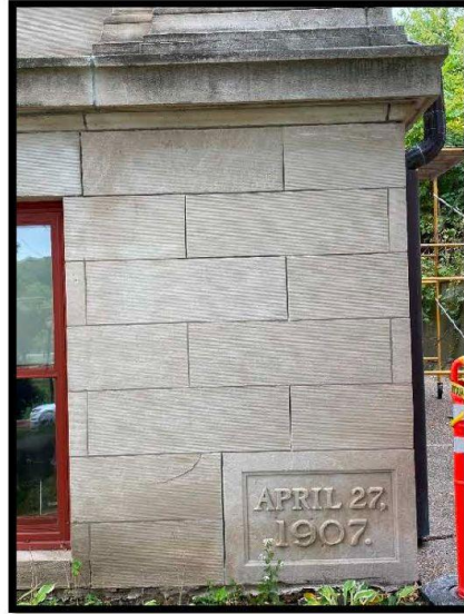
Stonework with Ground Out Joints and Prior to Power Wash
