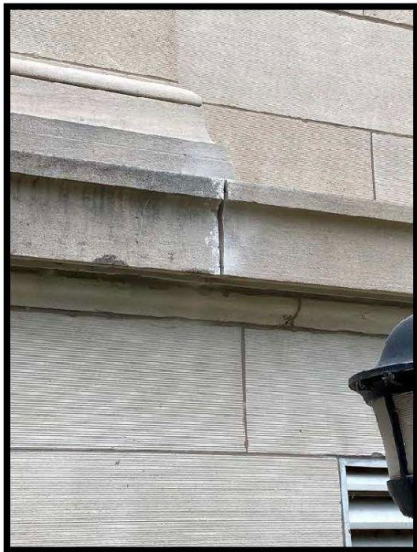
Joint Ground Out
