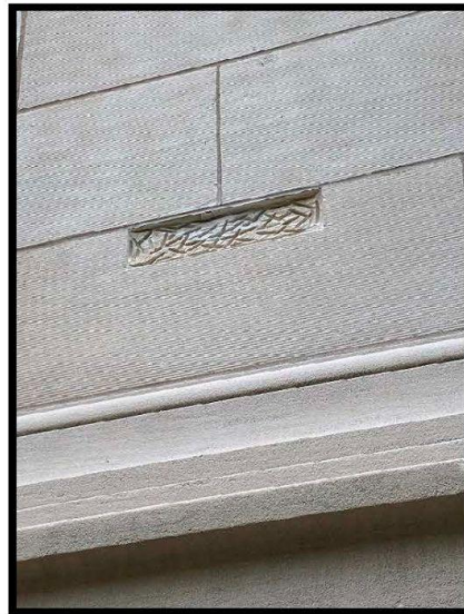
Stonework Preparation for Repair
