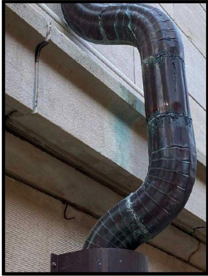
Downspout with Associated Green Staining
